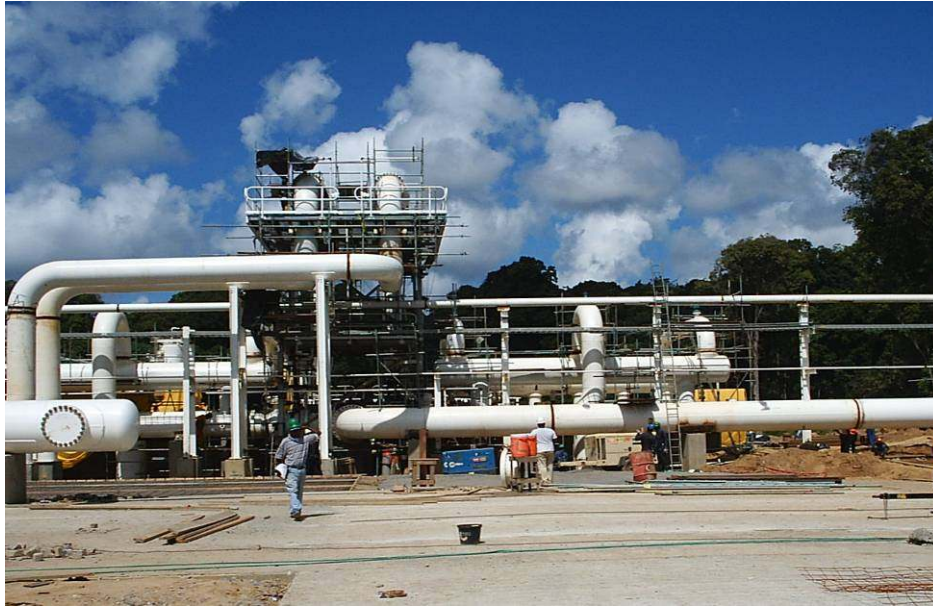
Figure 4: BUD Slug Catcher with Capacity to handle 3 Bcfd
