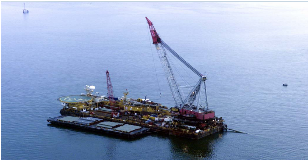
Figure 5: Snapshot of Pipe Laying Barge as it lays 36” pipes offshore
